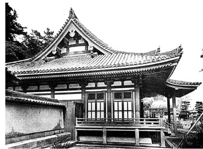
West Facade View
