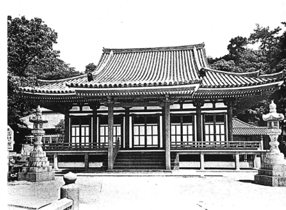
South (Front) Facade
