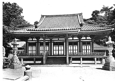
South (Front) Facade
