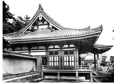
West Facade View
