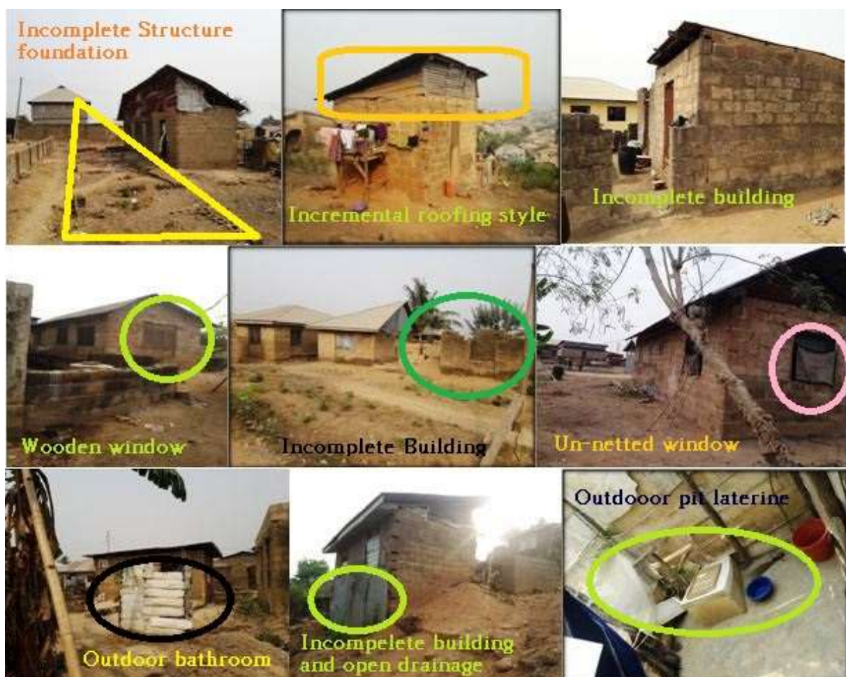
Figure 2. Pictorial Evidence and Visual Analysis of Sampled of Incremental Houses within the Sampled Enumerated Areas
