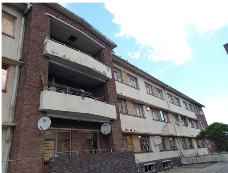
Figure 1. Cissie Gool House, Cape Town
