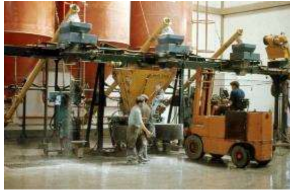
Figure 15. Factory: Storage of aggregates for the production of concrete and gypsum and automating gypsum production station
