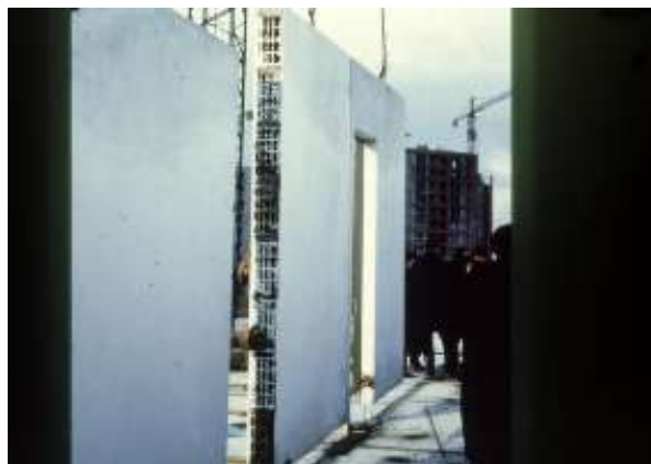
Figure 45. Assembly of panels on site
