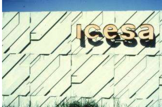
Figure 4. Prefabricated decorative panel at the entrance to the company complex
