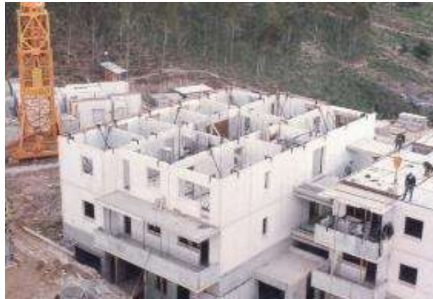
Figure 43. Assembly of the panels on site
