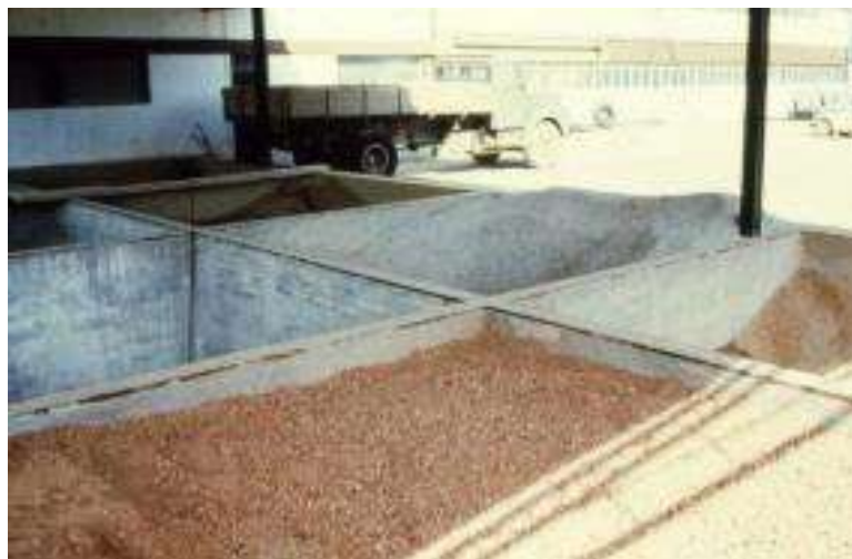
Figure 14. Factory: Storage of aggregates for the production of concrete and gypsum and Automating gypsum production station
