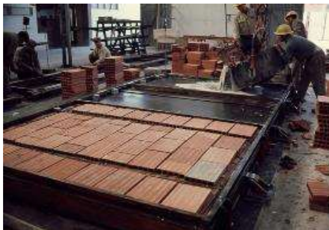
Figure 23. Partition wall panels and dividing panels with ceramic tiles as finishing
