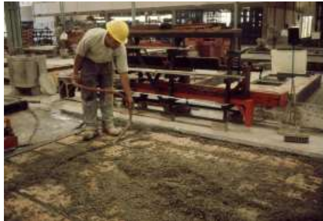
Figure 27. Slab panels and concrete vibration at reinforcement ribs
