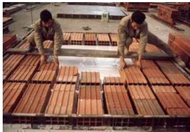
Figure 26. Slab panels and concrete vibration at reinforcement ribs
