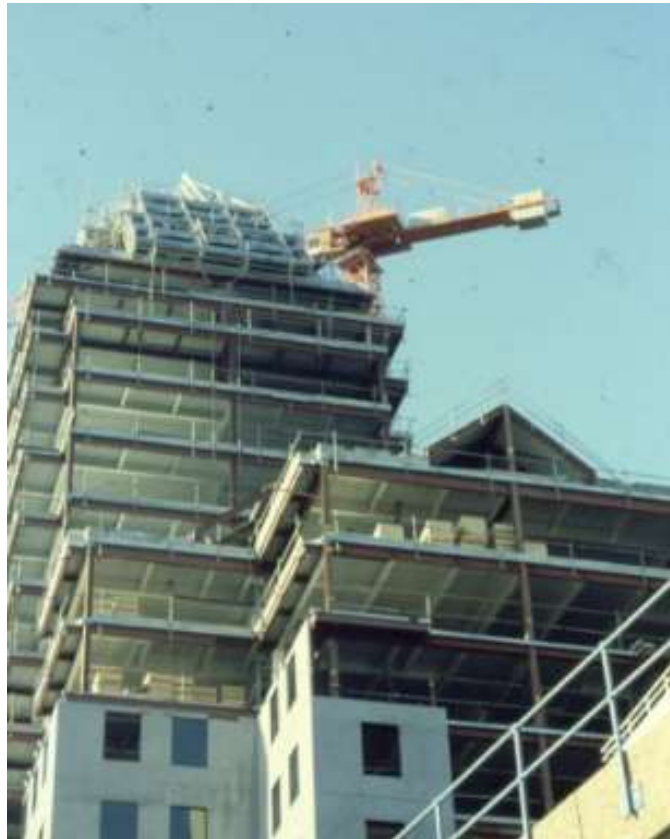
Figure 2. Partial prefabrication of exterior walls – conventional metallic structure
