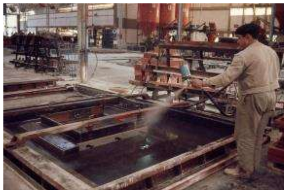
Figure 17. Factory: General view of the factory – metallic horizontal moulds, and Lubrication of the bottom of the mould in order to facilitate demoulding
