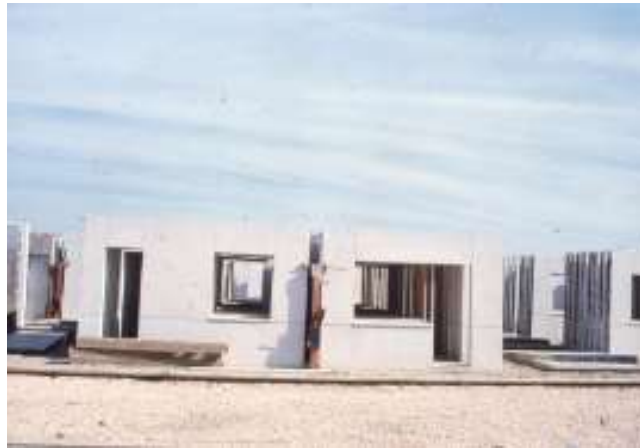
Figure 30. Exterior panels storage areas
