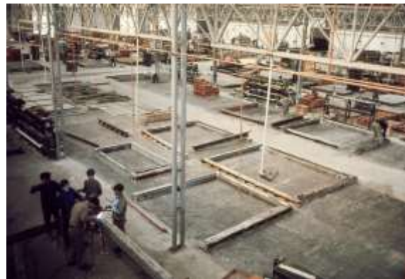
Figure 16. Factory: General view of the factory – metallic horizontal moulds, and lubrication of the bottom of the mould in order to facilitate demoulding
