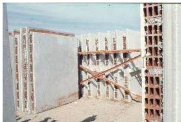
Figure 29. Exterior panels storage areas
