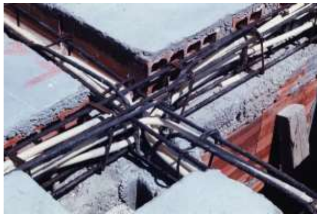
Figure 44. Assembly of the panels on site
