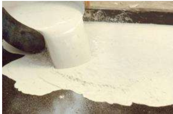
Figure 18. Gypsum plaster leaking into the mould
