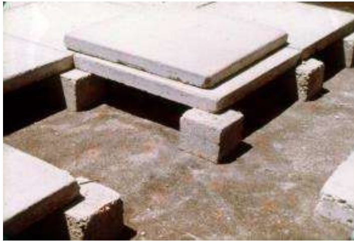
Figure 49. Roof protection paving slabs
