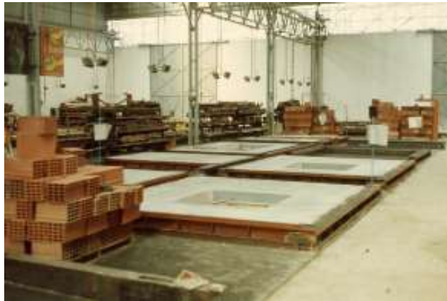
Figure 21. Factory: Concrete leakage and resistant exterior walls
