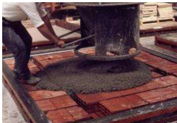
Figure 20. Factory: Concrete leakage and resistant exterior walls
