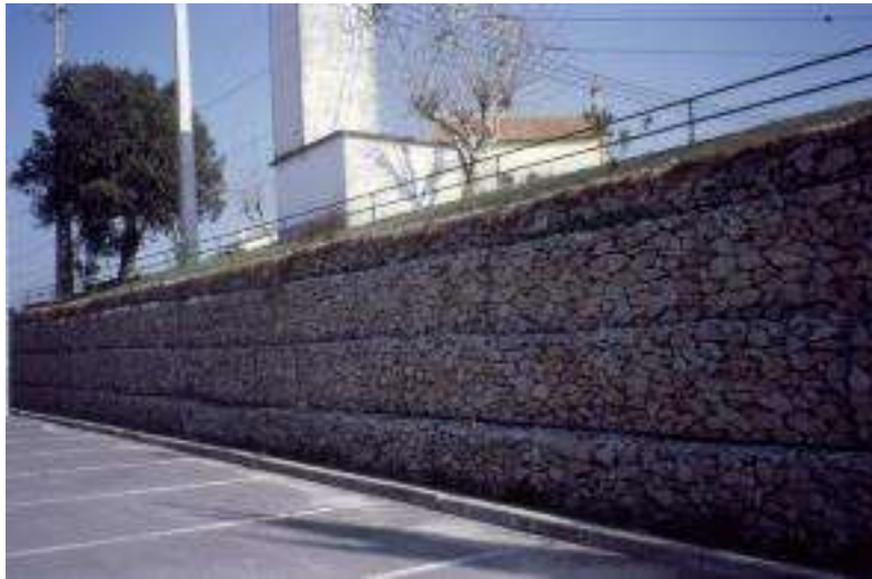
Figure 52. Gabion retaining wall
