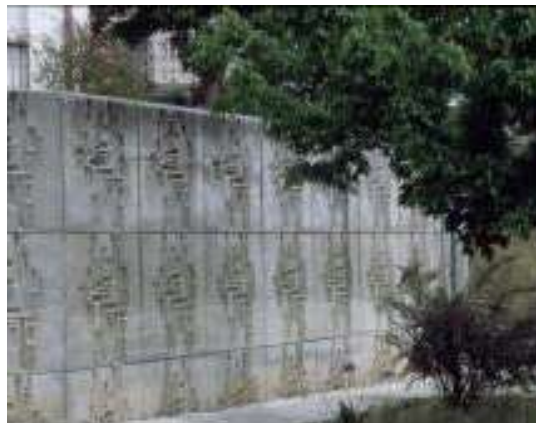
Figure 51. Retaining wall with prefabricated panels of moulded concrete
