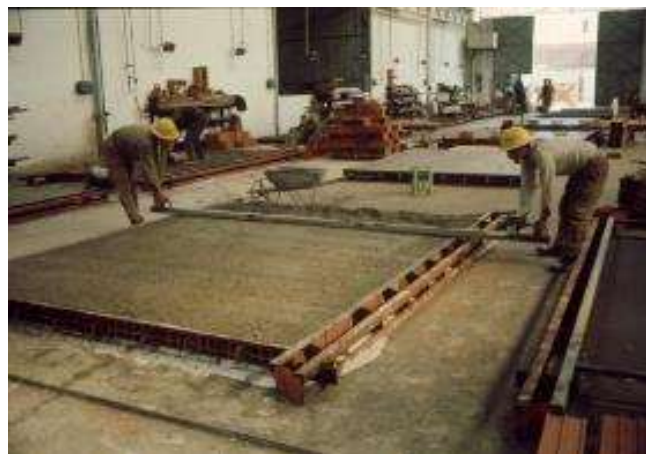
Figure 28. Regularisation of the concrete layer of the slab panel
