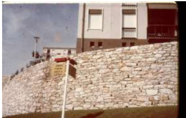
Figure 50. Retaining stone walls without mortar, and streets signage
