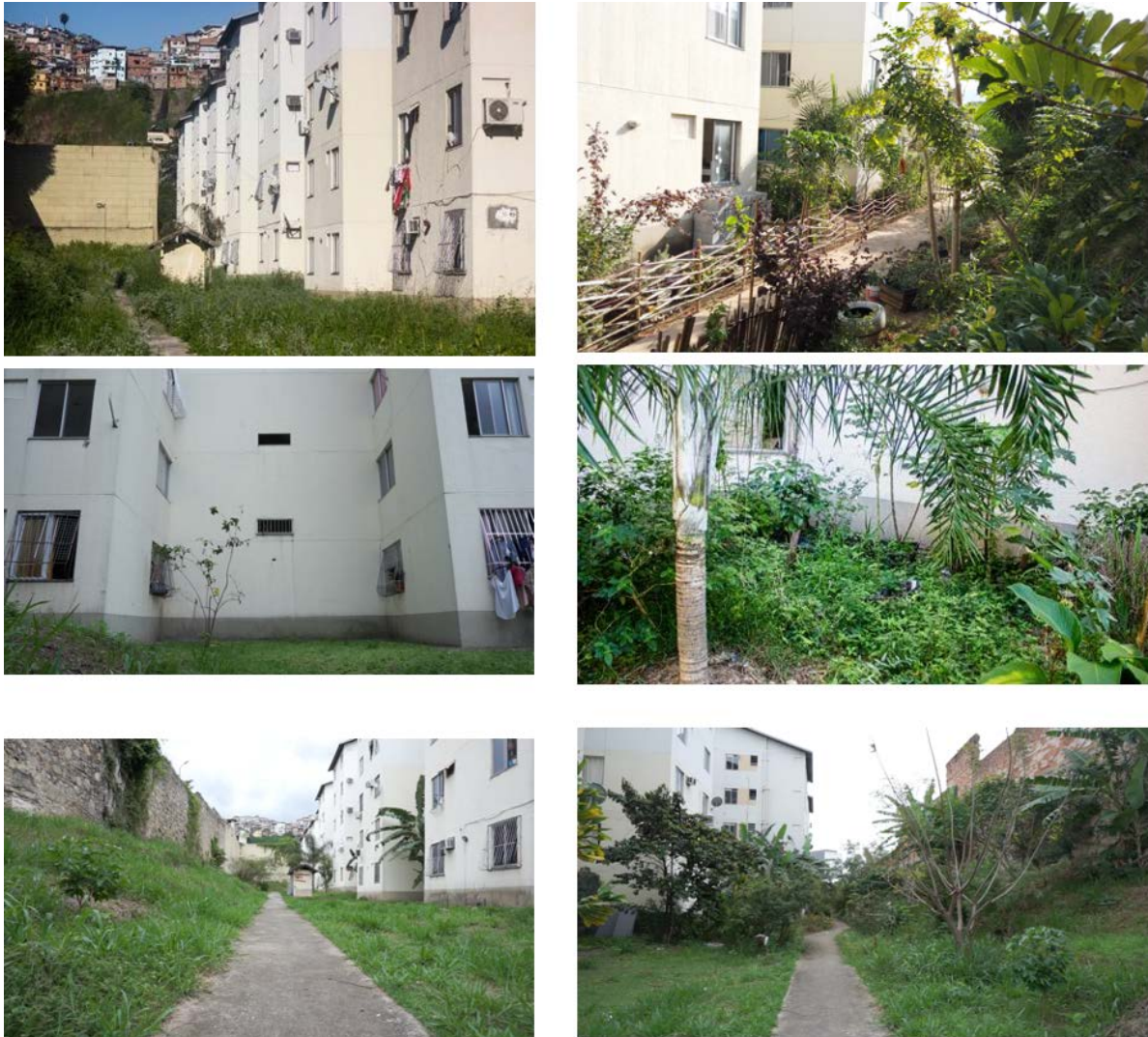
Figure 9. Surroundings of most buildings in the condominium (left) and contrast with the area of the Dja Guata Porã Garden (right)
