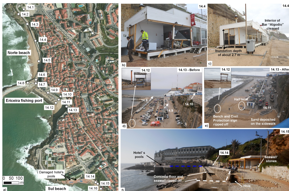
Fig. 6 – Field survey at Ericeira : a) Framework; b) Algodio bar destroyed; c) Bar and road cleaned from debris; d) and e) Point 14.13 before and after the storm; f) Damage at Sul beach.
