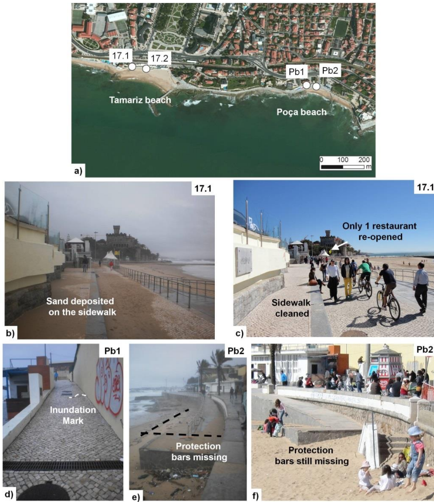
Fig. SM 7 – Field survey at Tamariz and Poça beaches, Estoril: a) Framework; b) Sand deposited on the sidewalk; c) Sidewalk cleaned; d) Inundation mark; e) Protection bars ripped off; f) damage still visible.
