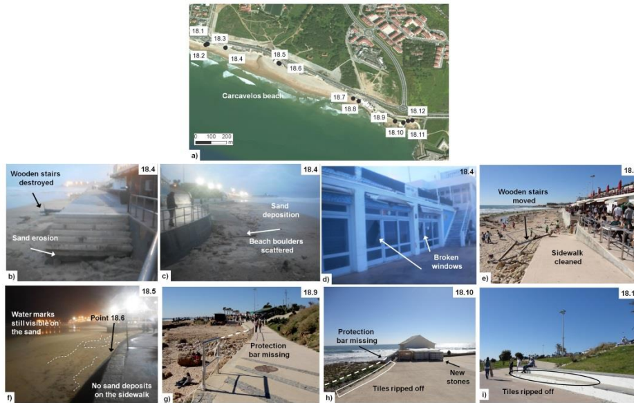
Fig. SM 8 – Field survey at Carcavelos beach: a) Framework; b) Erosion at the base of stairs; c) sand and boulders deposited; d) restaurants damaged; e) sidewalk cleaned, but damage was still visible; f) inundation marks at the beach; g) Protection bars still missing; h) Protection bars still missing and tiles ripped off; i) Tiles of the sidewalk ripped off.
