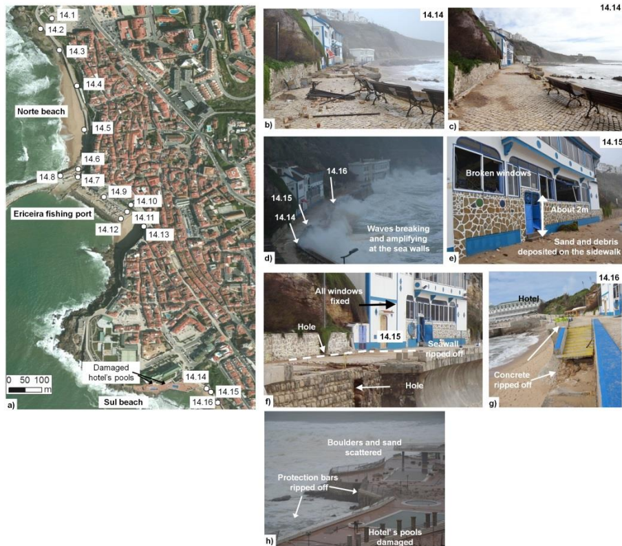
Fig. SM 6 – Field survey at Sul beach, Ericeira: a) Framework; b) damages on the Sul beach sidewalk. Photo by AZUL; c) sidewalk cleaned from debris; d) Sea waves hitting the Sul beach. Photo by AZUL; e) Damage on a restaurant. Photo by AZUL; f) Sea wall ripped off; g) Concrete structures ripped off; h) Damage on the hotel’s pools. Photo by AZUL.
