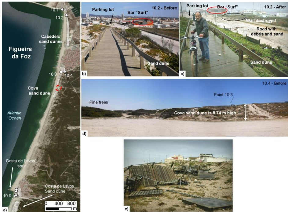
Fig. SM 3 – Field survey at Figueira da Foz: a) Framework; b) Cabedelo sand dune before the storm; c) Cabedelo sand dune after the storm. Photo taken by Pedro A. Cruz; d) Cova sand dune; e) Damage at Costa de Lavos. Photo taken by Pedro A. Cruz.
