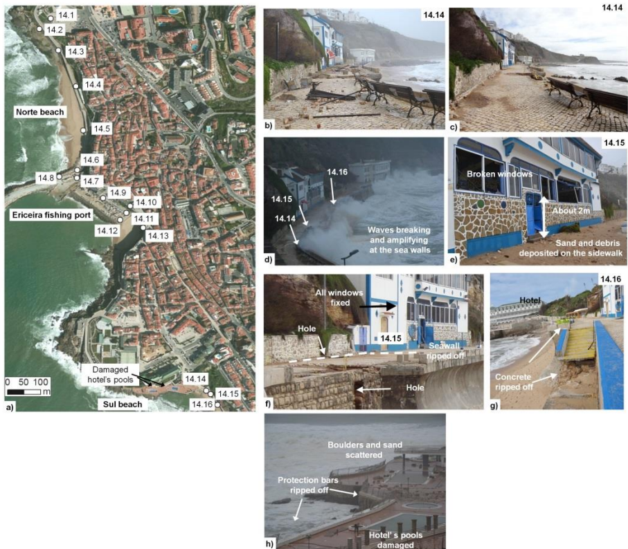
Fig. SM 6 – Field survey at Sul beach, Ericeira: a) Framework; b) damages on the Sul beach sidewalk. Photo by AZUL; c) sidewalk cleaned from debris; d) Sea waves hitting the Sul beach. Photo by AZUL; e) Damage on a restaurant. Photo by AZUL; f) Sea wall ripped off; g) Concrete structures ripped off; h) Damage on the hotel’s pools. Photo by AZUL.
