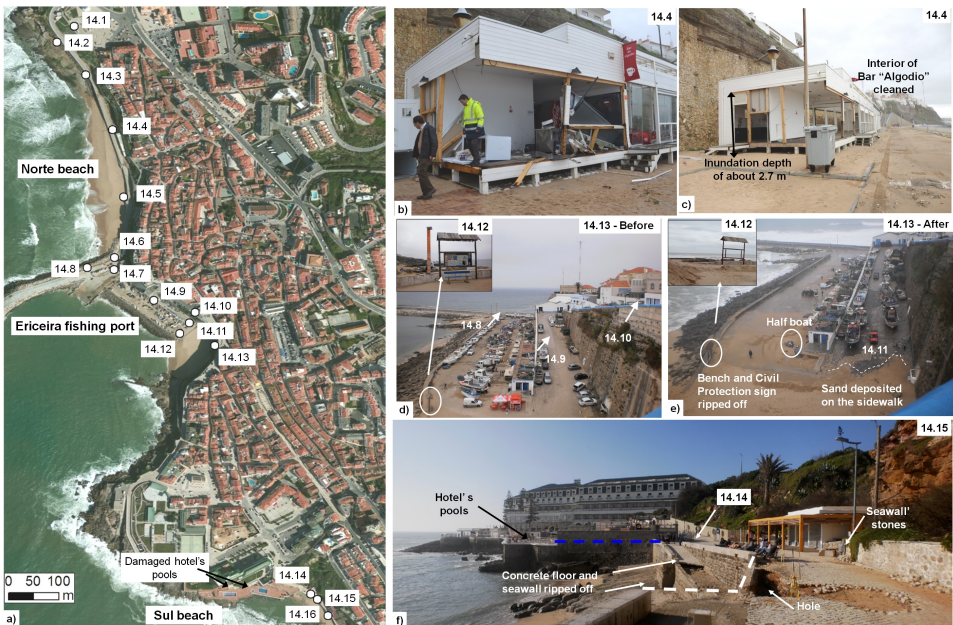
Fig. 6 – Field survey at Ericeira : a) Framework; b) Algodio bar destroyed; c) Bar and road cleaned from debris; d) and e) Point 14.13 before and after the storm; f) Damage at Sul beach.
