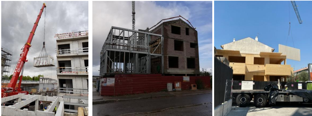
Figure 1 – Different prefabricated construction systems: (a) modular concrete construction; (b) LSF construction; (c) CLT panel construction
