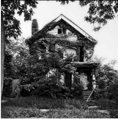
ONE OF DETROIT'S ABANDONED AND OVERGROWN HOUSES, [P] CAROL MARTIN
