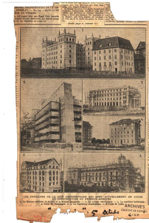
Figure 1. The various halls of residence of the Cité Universitaire under construction. Fragment of a newspaper report published in the French press. Unknown origin (circa 1932). In the photographs, the stage of the works on the Colegio de España (Spanish), the maison de la suede (Swedish), the Fondation Hellénique (Greek), Fondation Danoise (Danish), the Maison des Étudiants Arméniens (Armenian) and, finally, the Maison de Cuba (Cuban) may be observed (ACE, 148/1).
