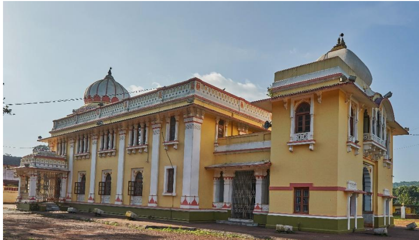
Figure 4. Rebuilt Vithal temple of Sanquelim
