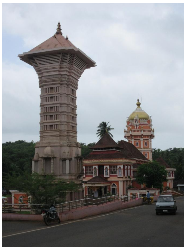
Figure 11. Kapileshwar after rebuilding Source: Photograph by the author
