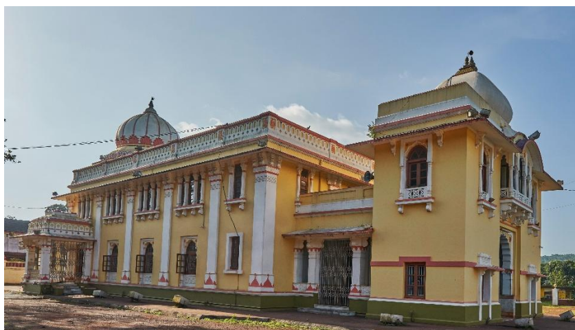
Figure 4. Rebuilt Vithal temple of Sanquelim
